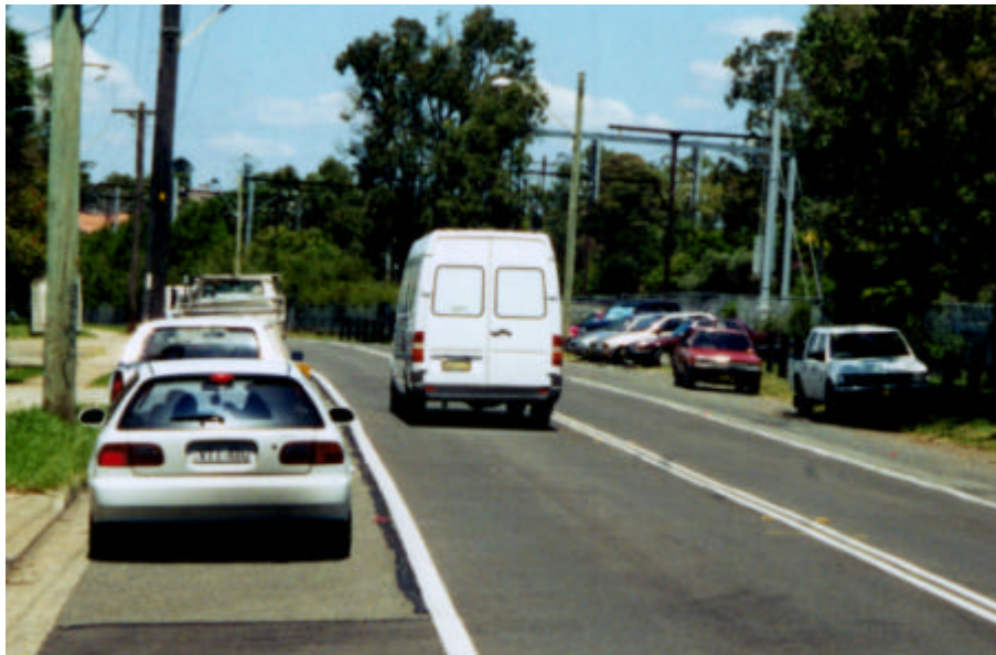
Wentworth Avenue Pendle Hill looking east
